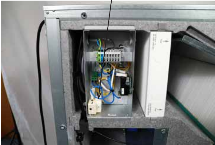
Built-in electric heating surface in ECO 400 XL
