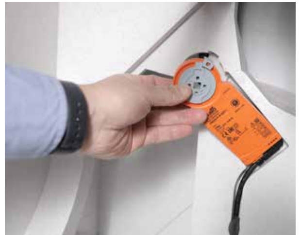
Remove bypass actuator
