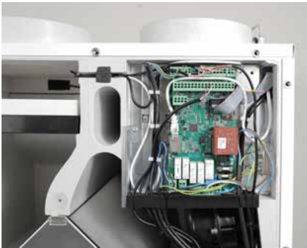
Remove control board
