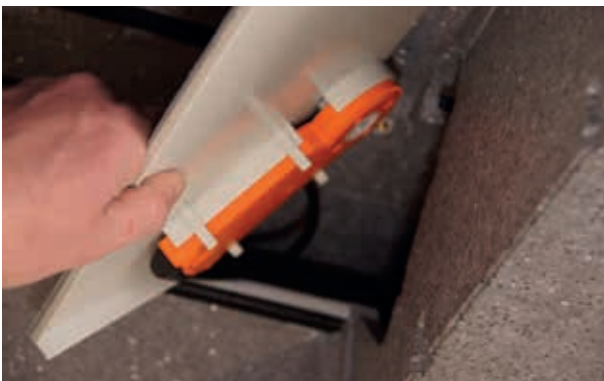
Remove bypass actuator
