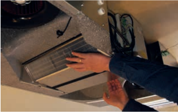
Remove heat exchanger
